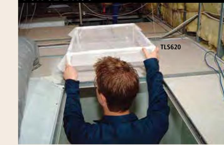
**PIG** Ceiling Tile Leak Diverters install in office areas for low-profile protection that won't get in your way.
